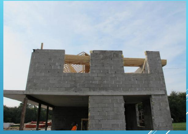
ROOF DECKING STARTED AND THE PRECAST ROOFING WAS REMOVED FOR THE 2<sup>ND</sup> & 3<sup>RD</sup> FLOOR ADDITION
